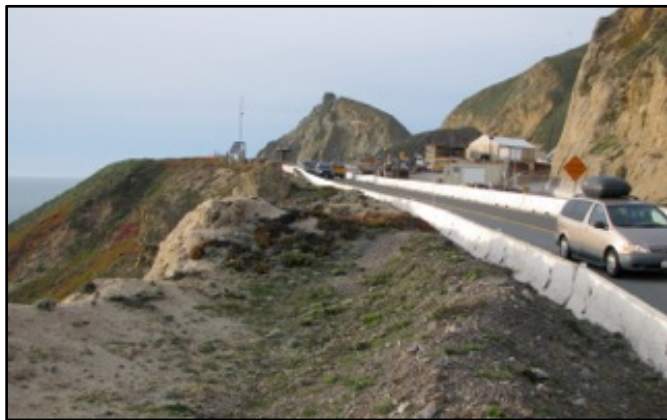
Issue: Fill and retaining wall needed
