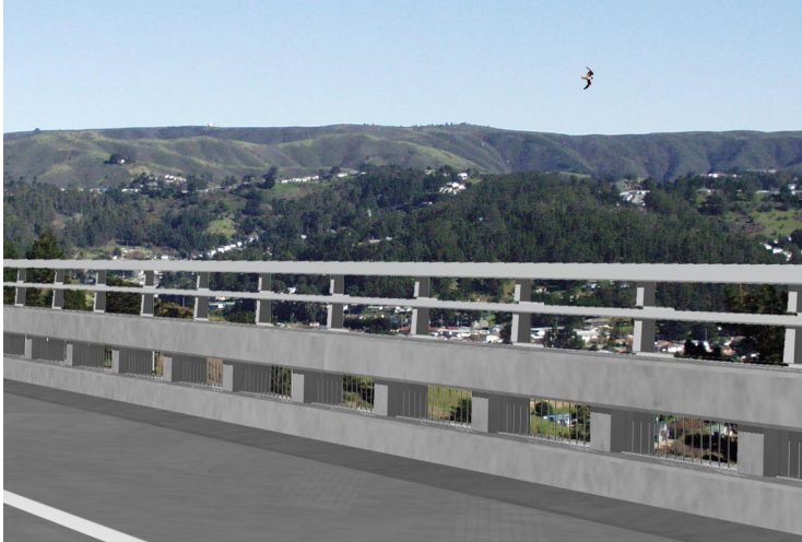
Figure 3.4.1b: Type 80 Bridge Barrier with Pedestrian/Bicyclist Railing
