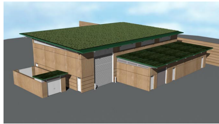
(a) OMC Building with a Sod Roof
