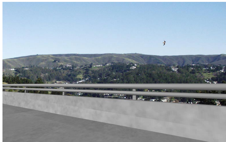
Figure 3.4.1a: Standard Solid Bridge Barrier with Pedestrian/Bicyclist Railing
