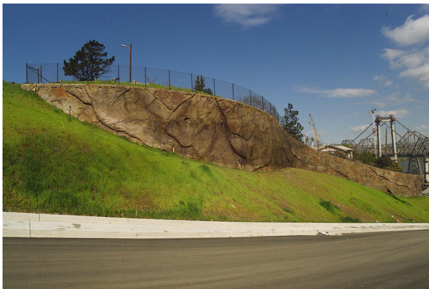
Figure 3.2c Retaining Wall along Route 80 in Crockett
