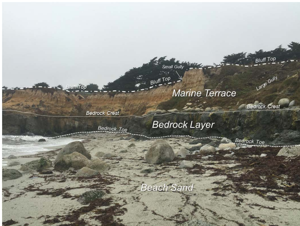
Figure 2 Photograph of site on beach looking north, showing the stratified geology of the bluff
