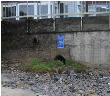
Capistrano Outfall Pipe
