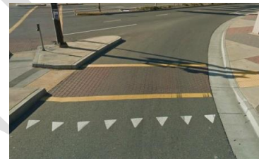
Figure 5: Advance Yield Markings at a Pedestrian Crossing
