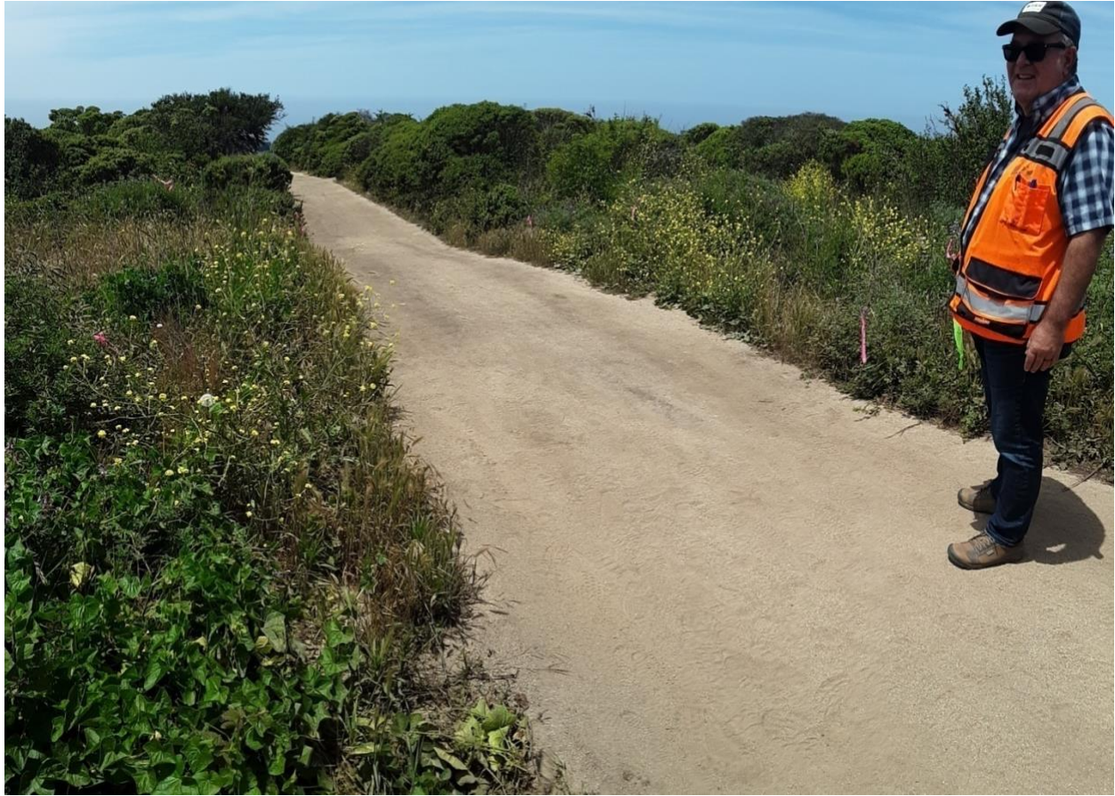
Figure 8: The access road narrows to ten feet in width at elevations above station 100 with butterfly host plants growing along the edges. These lupines will be impacted when the roadway is widened to 12 feet on the straightaways and 15 feet on the corners.
