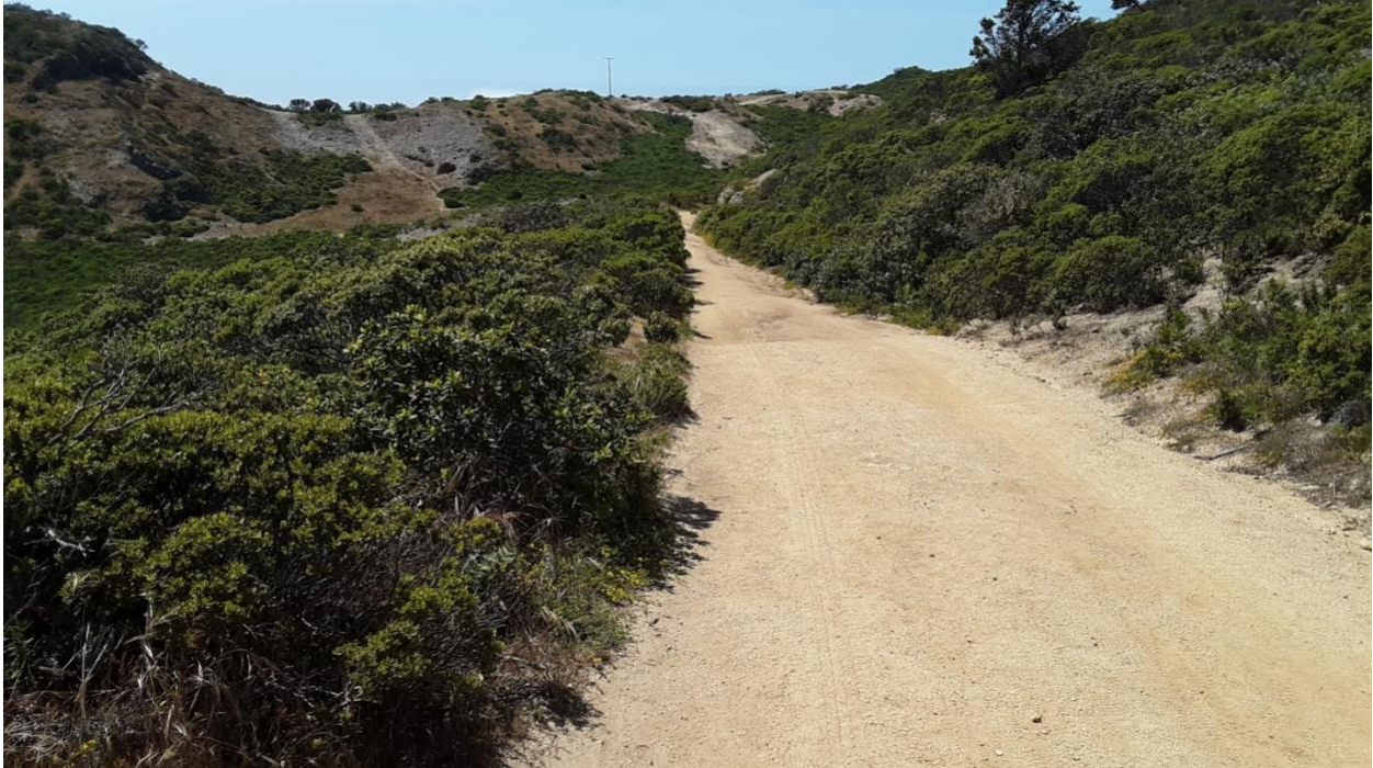
Figure 17: View south of Station 184 at mile 3.5 where the 10-foot roadway would need to be widened to 20 feet to meet the requirements of the proposed fire turnout. This would require extensive vegetation removal.
