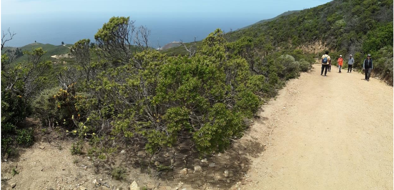
Figure 6: The Mitigated Negative Declaration states that new turnouts will occur on flat areas yet the 1st proposed turn out at Station 96+00 will occur on a 12% slope of decomposed granite. The roadway is currently 15 feet wide with a deep ditch on the northern edge to capture runoff from the steep sided granite hillside. Construction of a new turnout will require the removal of 300 square feet of dense coastal scrub. A qualified biologist should conduct surveys for nesting birds, special status plants and butterfly host plants prior to the cut and fill required to form the turnout.
