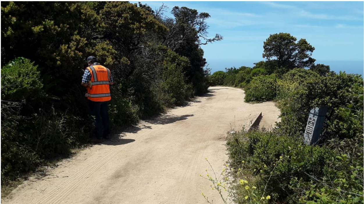
Figure 10: Facing west, view of the 3rd proposed turn out located at station 136+00 and at the top of the pedestrian trail to San Pedro Park in Pacifica. Construction of this turnout will require cut and fill and the removal of ~ 700 square feet of dense coastal scrub.
