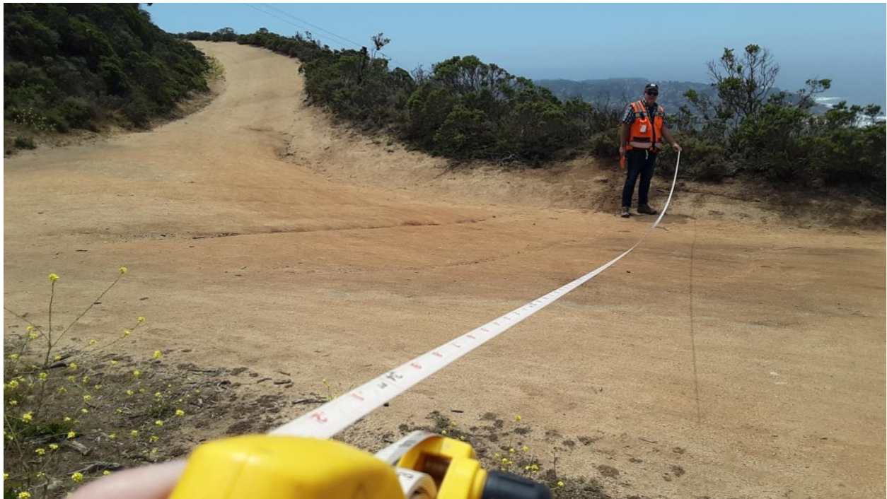
Figure 5: The existing utility clearing at station 81+00 has the dimensions (88' x 34') to be used as a fire turnout.
