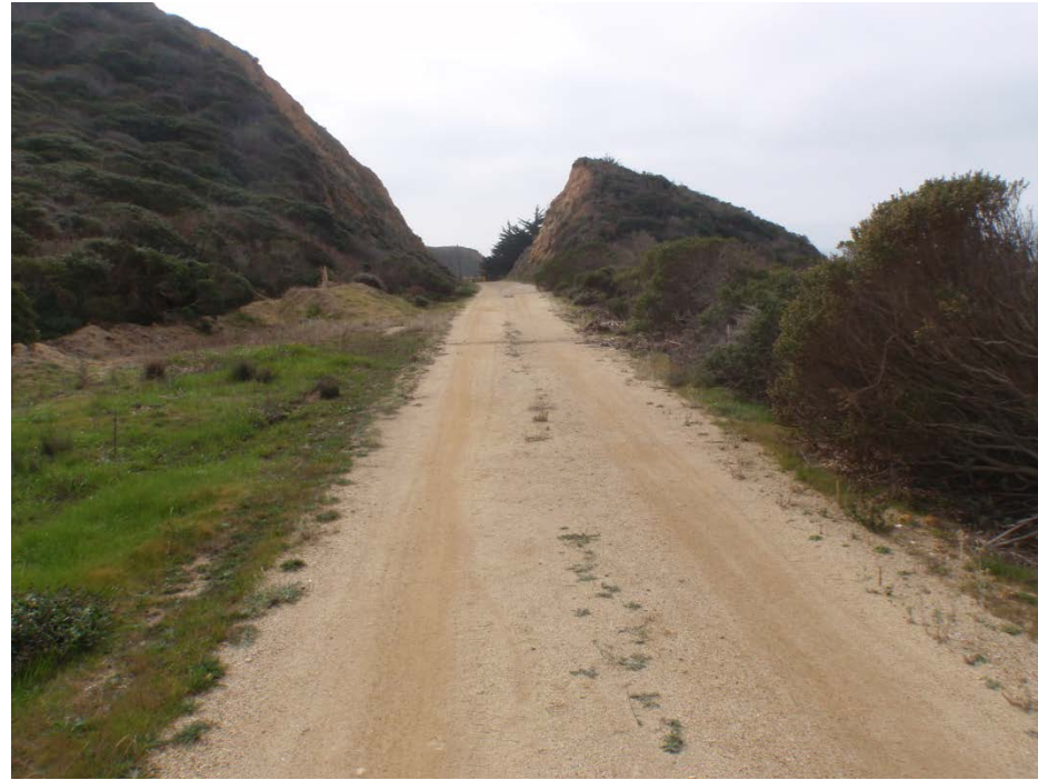
Existing Access Road (looking southwest)
