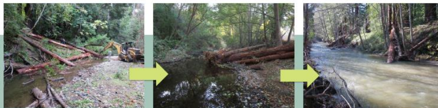
Secured log fisheries habitat structure installations
