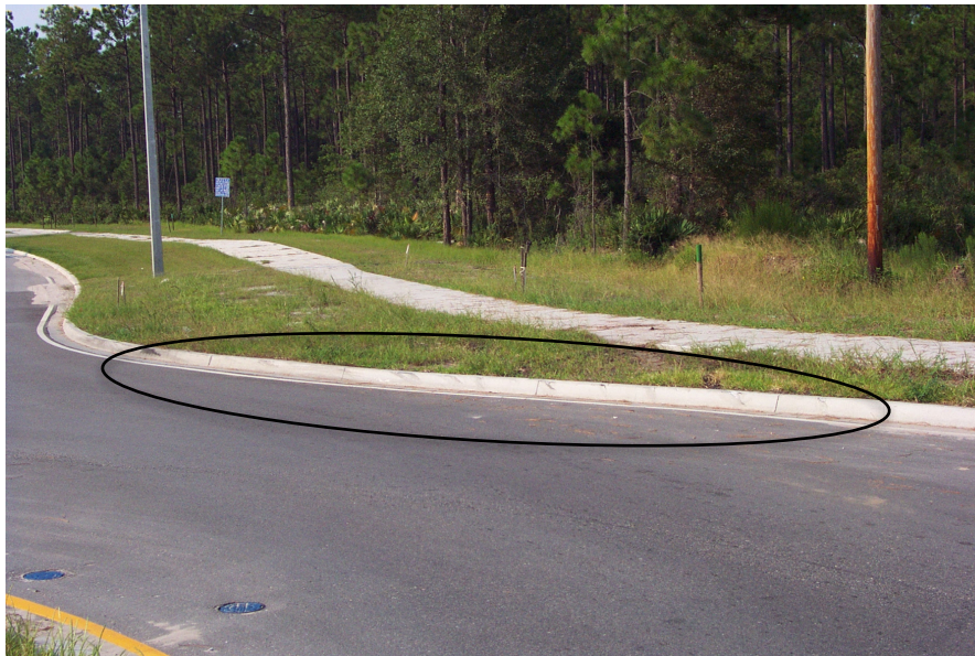
Figure 3. A roundabout with a fast entry speed and a low-speed exit showing many hits of the exit curb.
