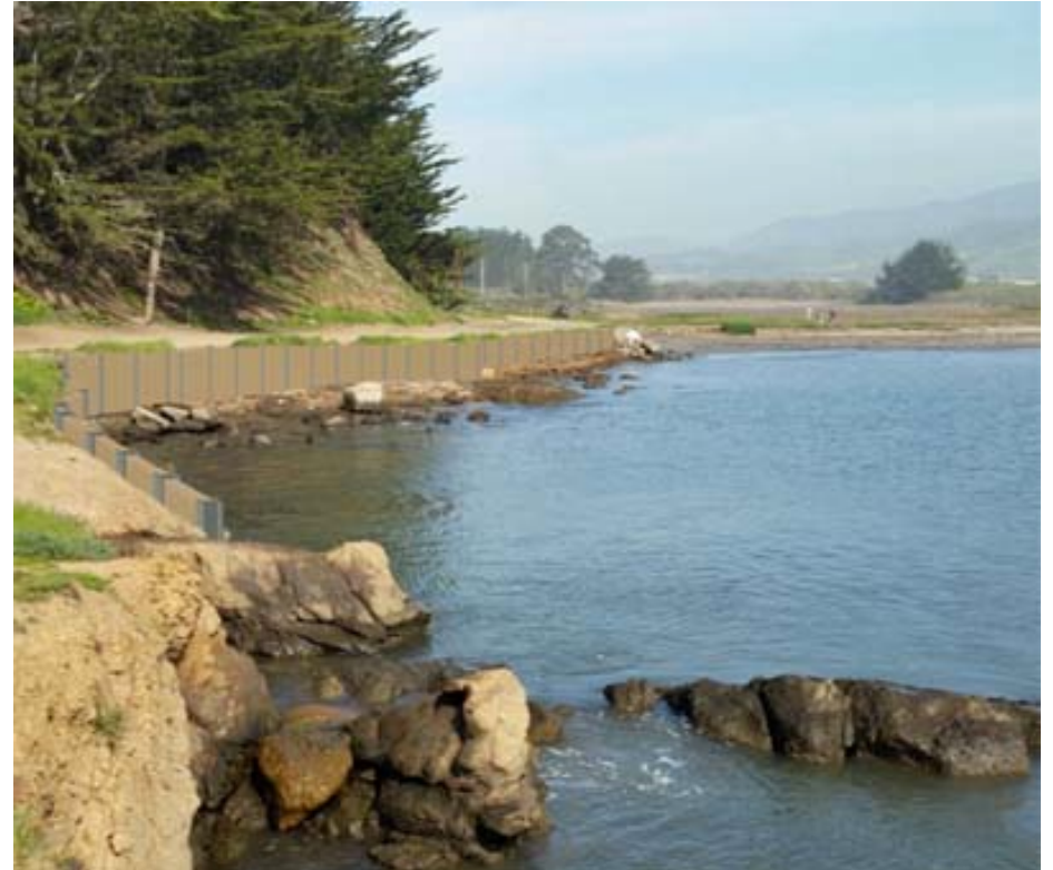
soldier pile wall simulation
