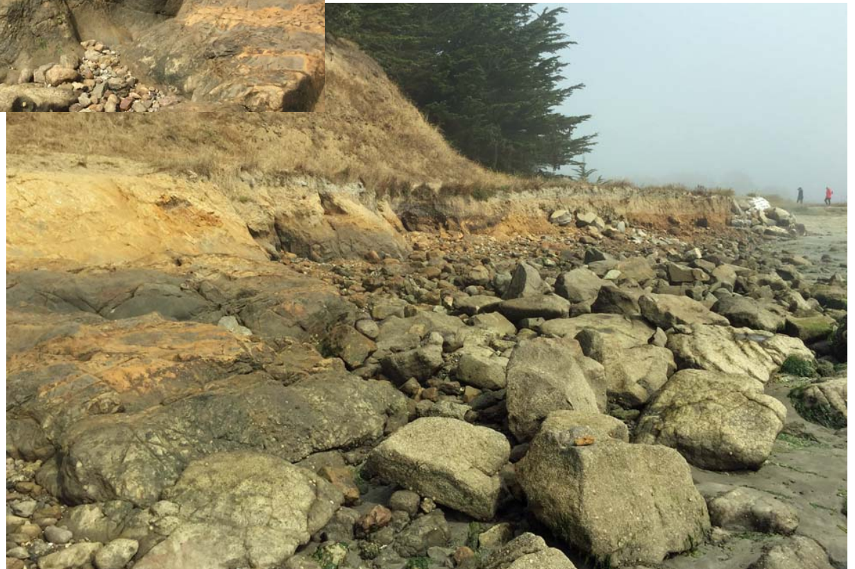
Looking north from bedrock outcrop toward culvert
