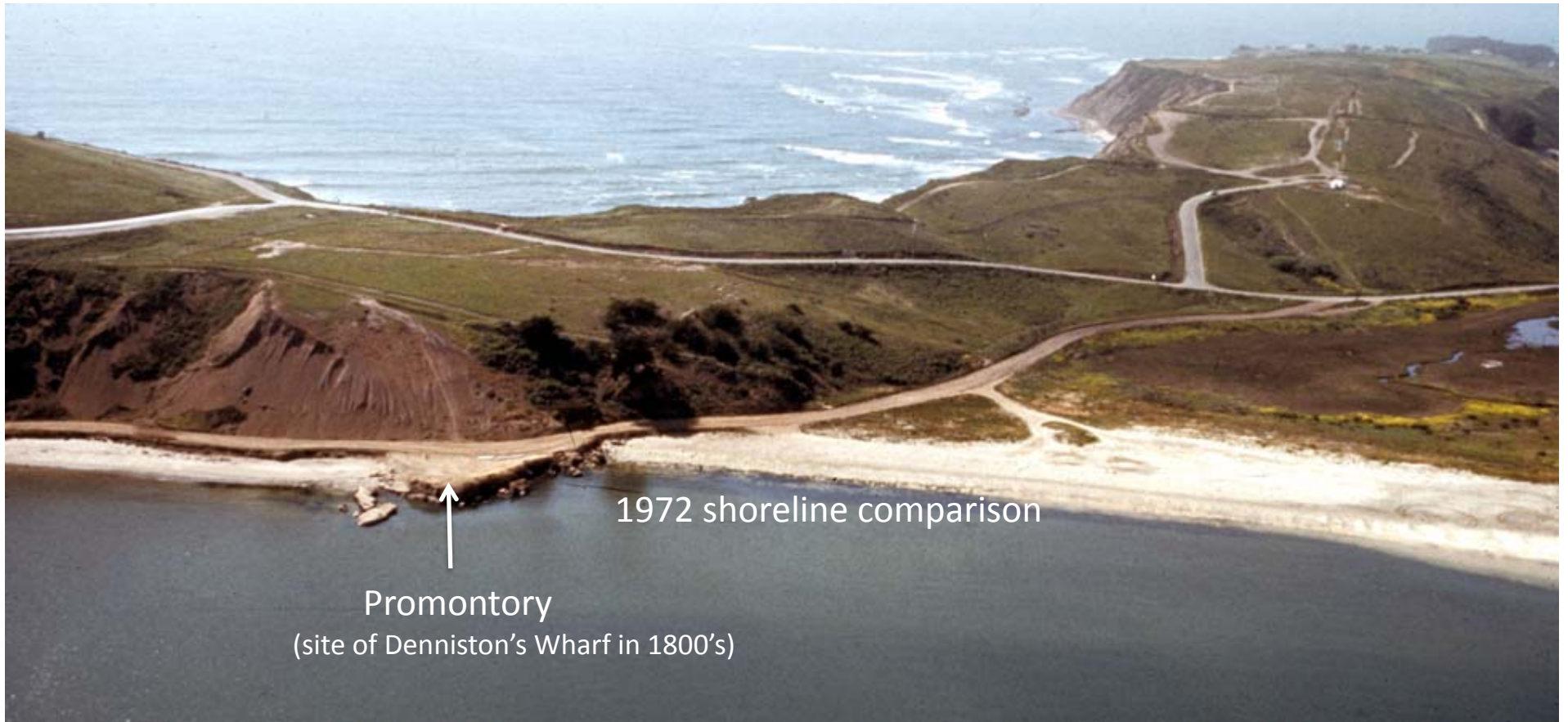
US Army Corps leveled and built the road out to Pillar Point to build the breakwater in 1959.
