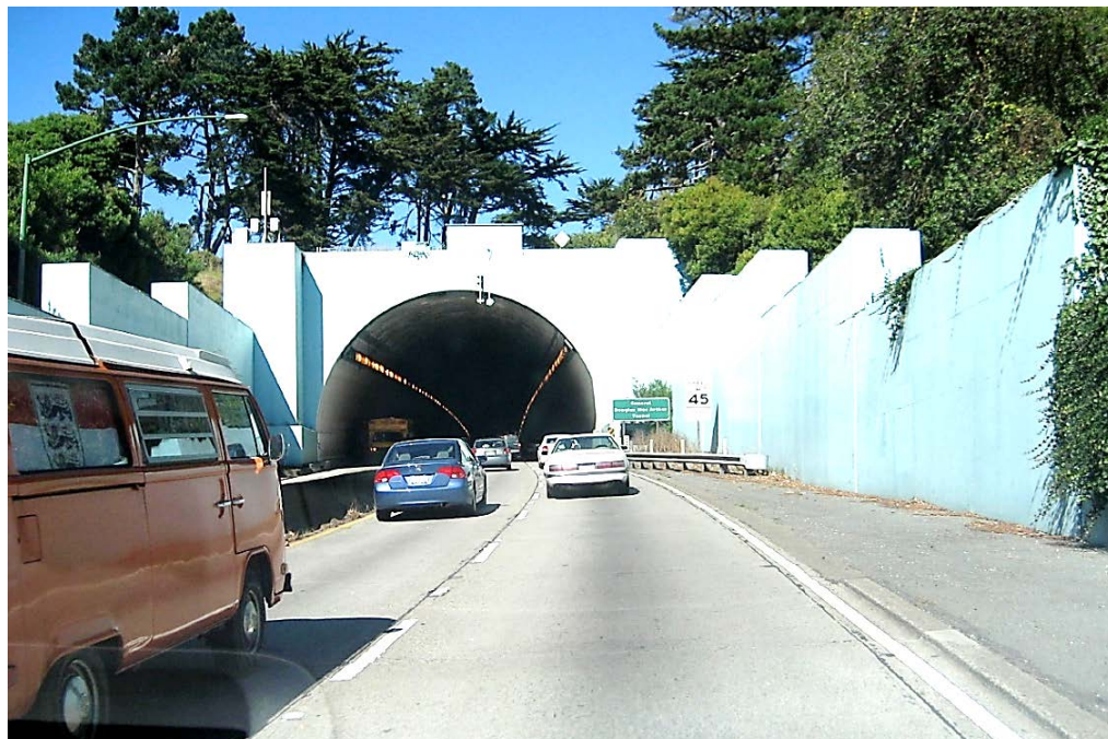
General MacArthur Tunnel, San Francisco Presidio
