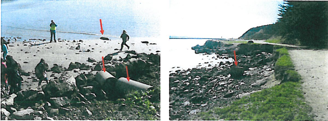
Photo 9 – Concrete rubble on beach, Sta 6+00
