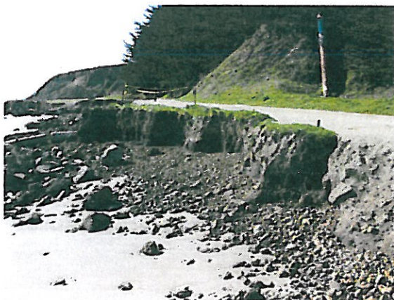
Photo 3 – Looking South, showing eroded areas encroaching into path, Sta 5+50 to 6+00
