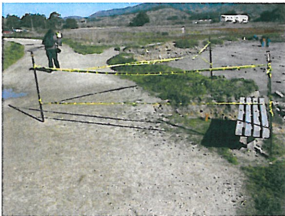
Photos 7 & 8 – Sta 6+00, showing severe erosion at stacked non-functioning culverts.
