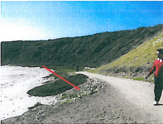
Photo 15 – Southern portion of path, taken from Sta 9+75. Eroded area indicated.
