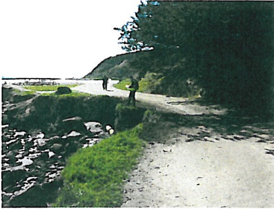
Photo 5 – Looking South, showing eroded areas encroaching into path, Sta 7+50 to 8+00
