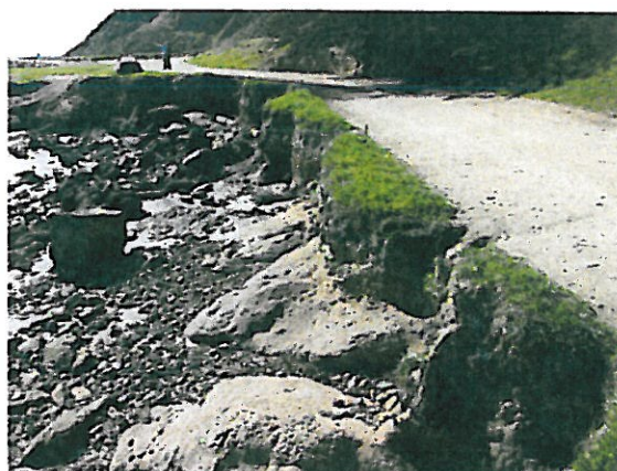
Photo 3 – Looking South, showing eroded areas encroaching into path, Sta 5+50 to 6+00
