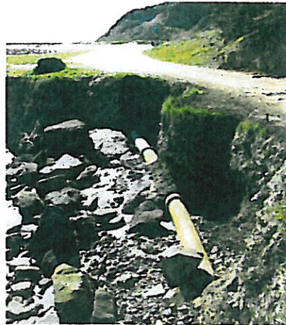
Photo 5 – Looking South, showing eroded areas encroaching into path, Sta 7+50 to 8+00
