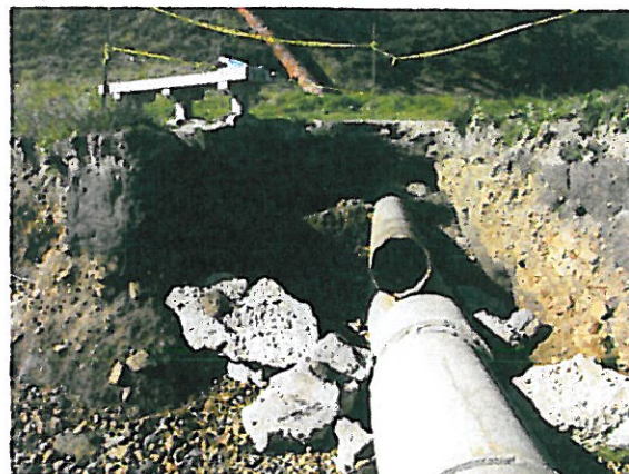
Photos 7 & 8 – Sta 6+00, showing severe erosion at stacked non-functioning culverts.
