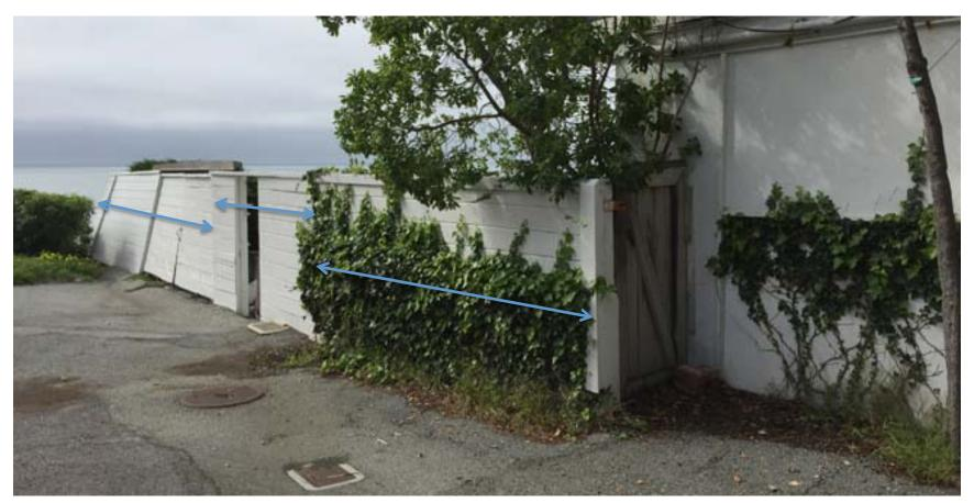
South fence section and double gates proposed for removal have failed and are leaning against the Cypress behind.
