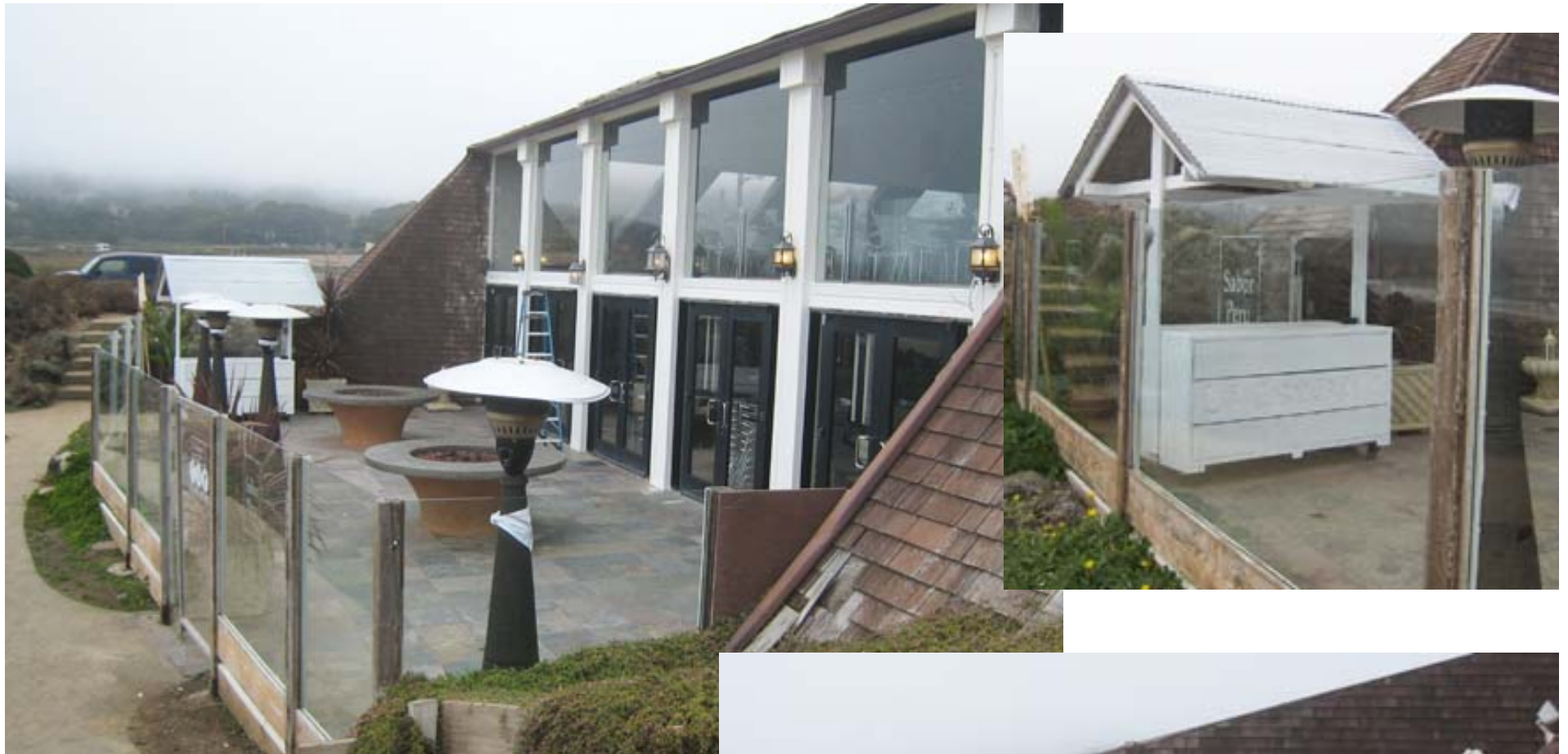
More bright white paint over formerly natural wood finish: bar shack, deck screen - painting in progress 9/19/14.
