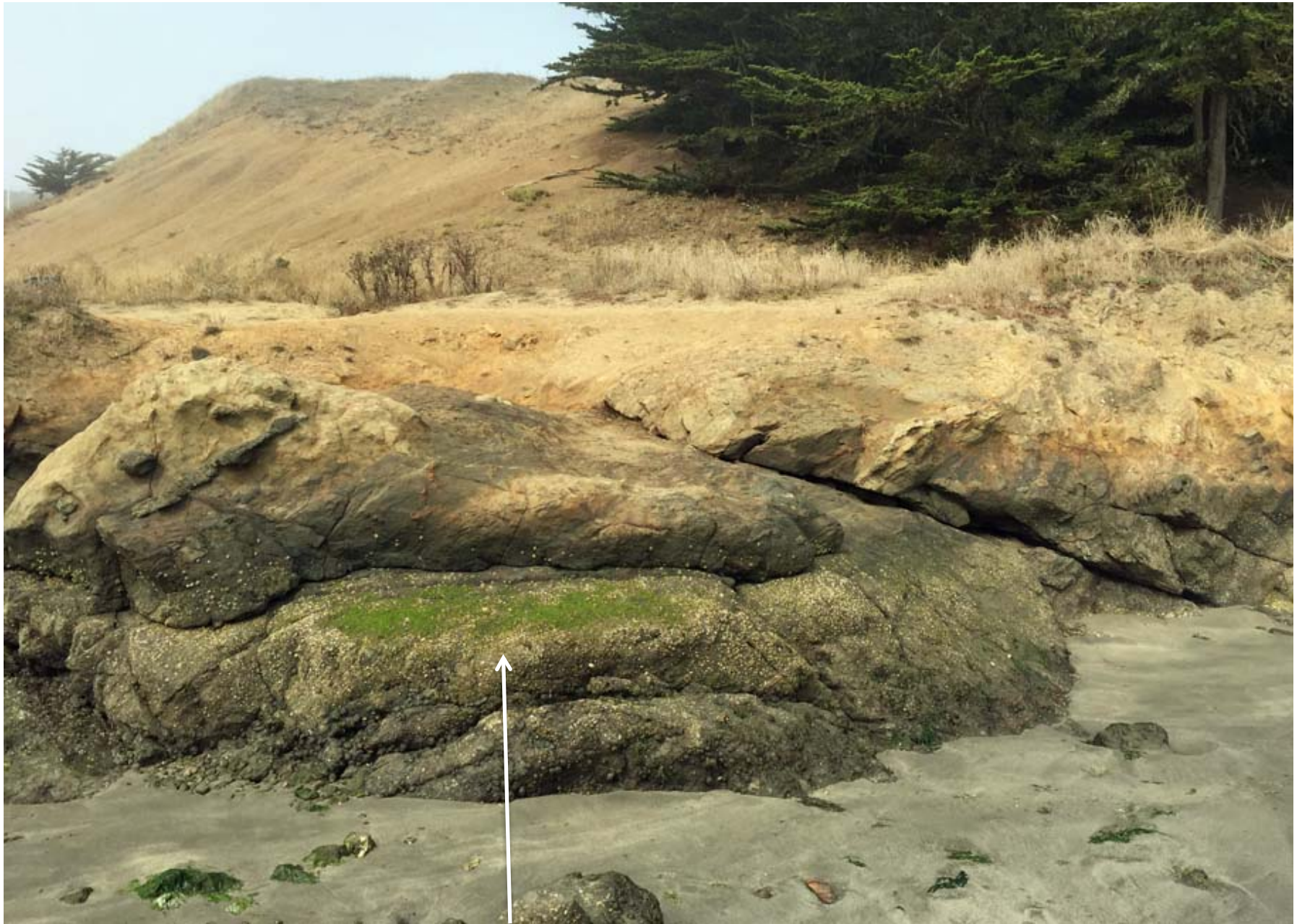
Natural bedrock at West Shoreline Trail – a model for sculpted shotcrete soil-nail wall
