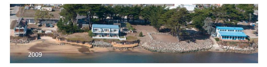
3-story 1993 house at Columbia, with unpermitted riprap in front. Tall narrow building towers over beach on substandard 25-ft-wide lot. This east-side view shows extensive erosion of parcels east of riprap.
