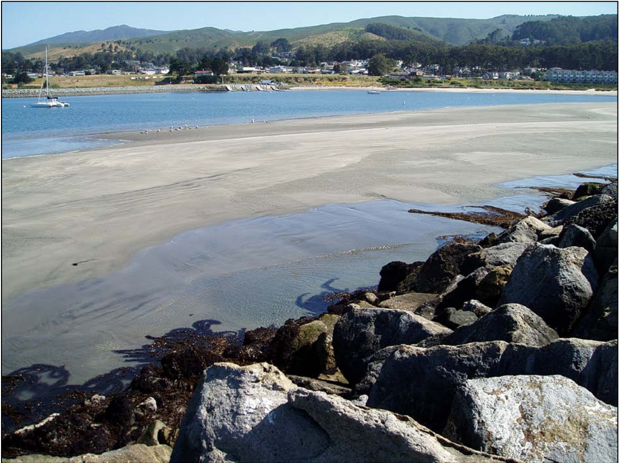
Figure 48. Photograph looking into Pillar Point Harbor showing surging of water through the east breakwater (Source: Craig Conner)
