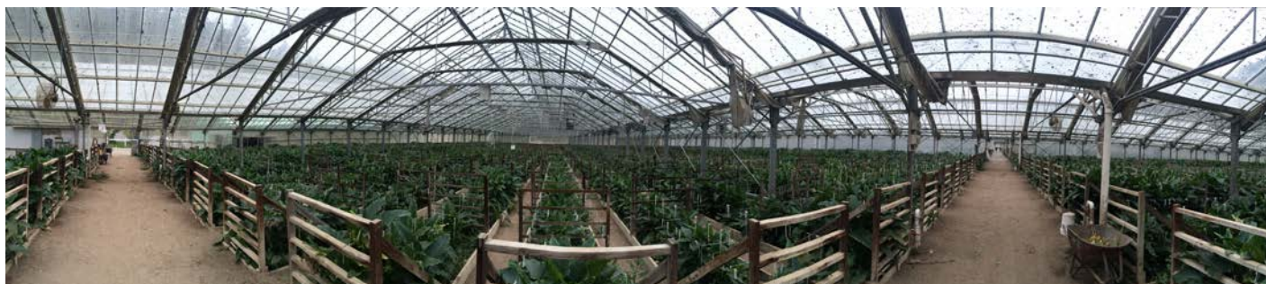
Photo 5: Pescadero Greenhouse Panorama (265,000 Square Feet Facility)
