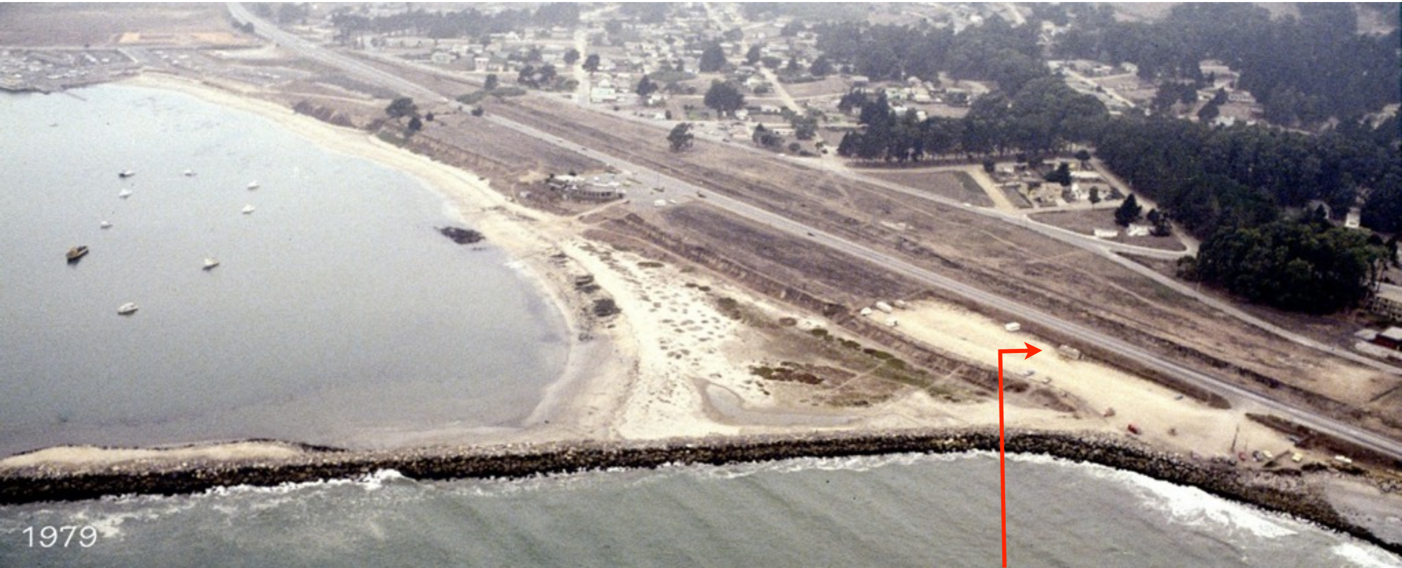
Surfer's Beach Restroom
