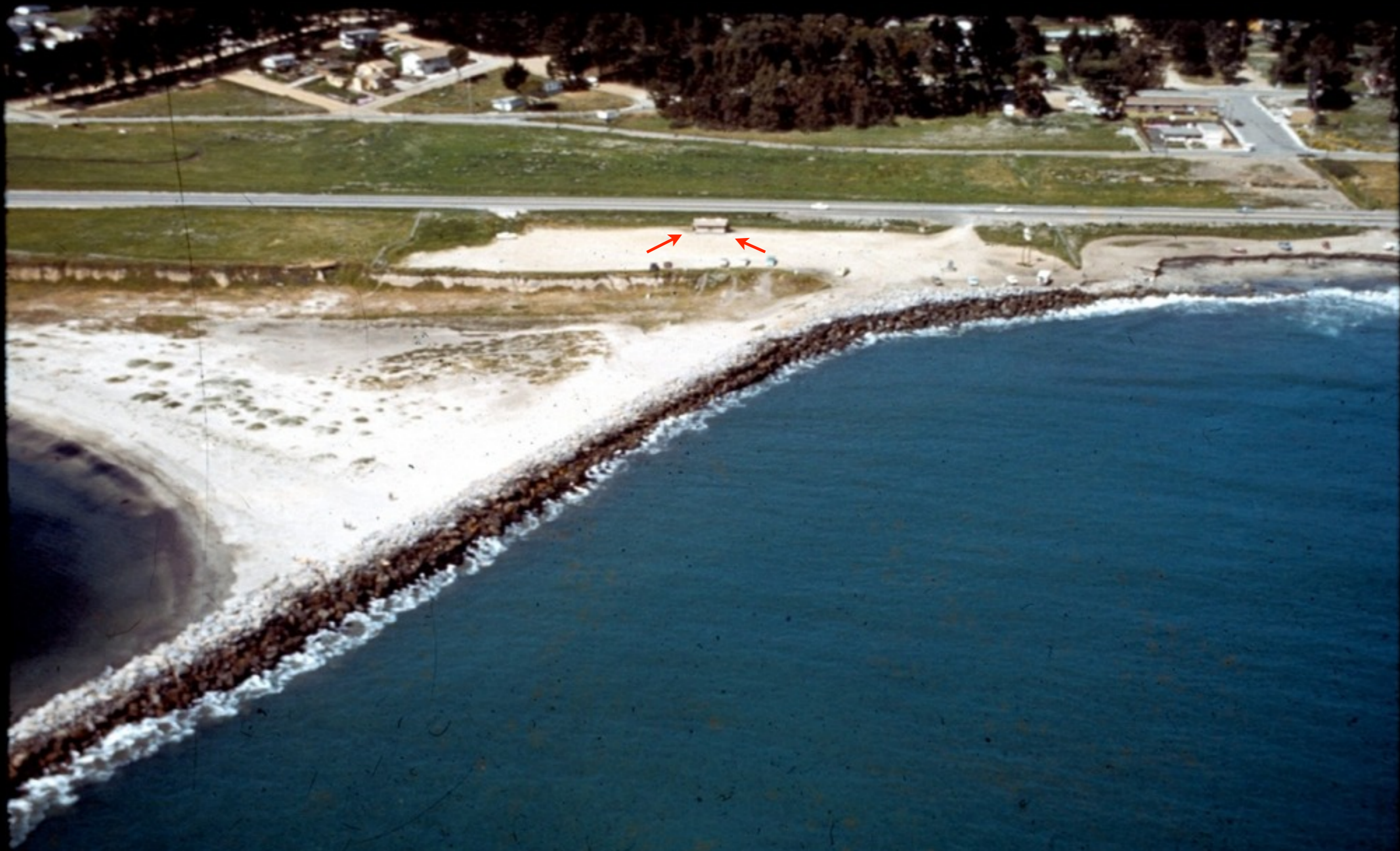
Surfer's Beach public restroom and public parking 1972
