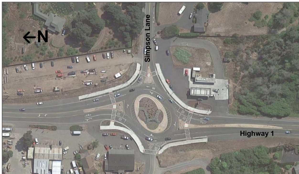
Figure 5: Multi-Lane Roundabout at Highway 1 and Simpson Lane, Fort Bragg, CA
