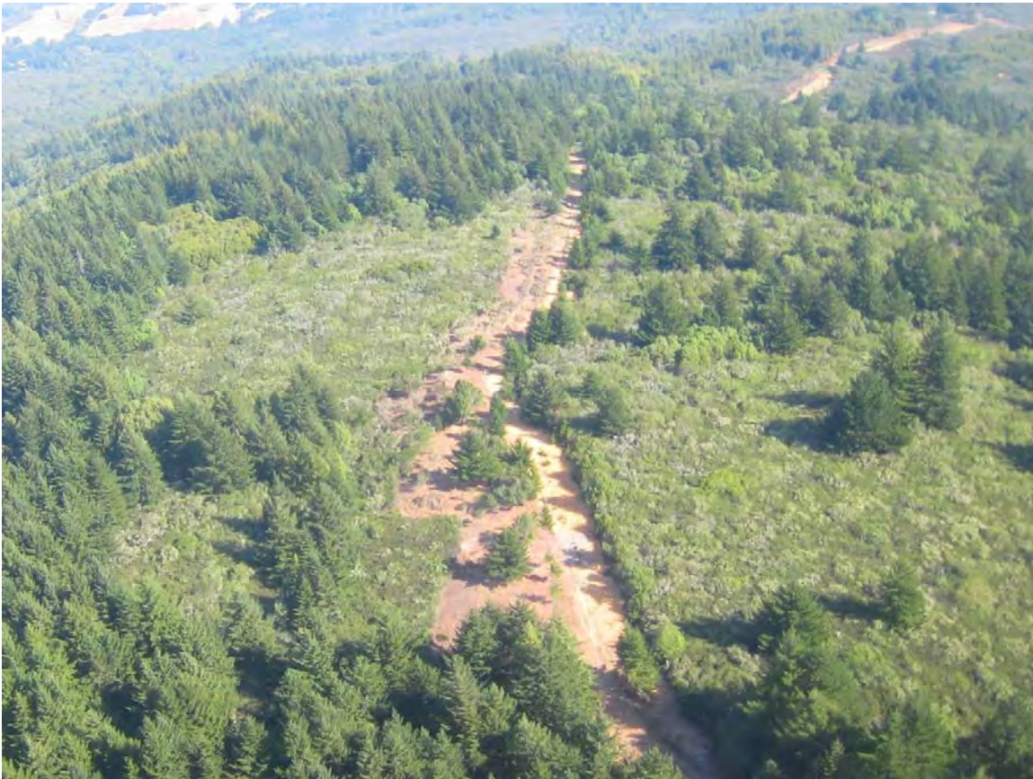
Crystal Springs Southern Fuel Break in San Mateo County. 2008
