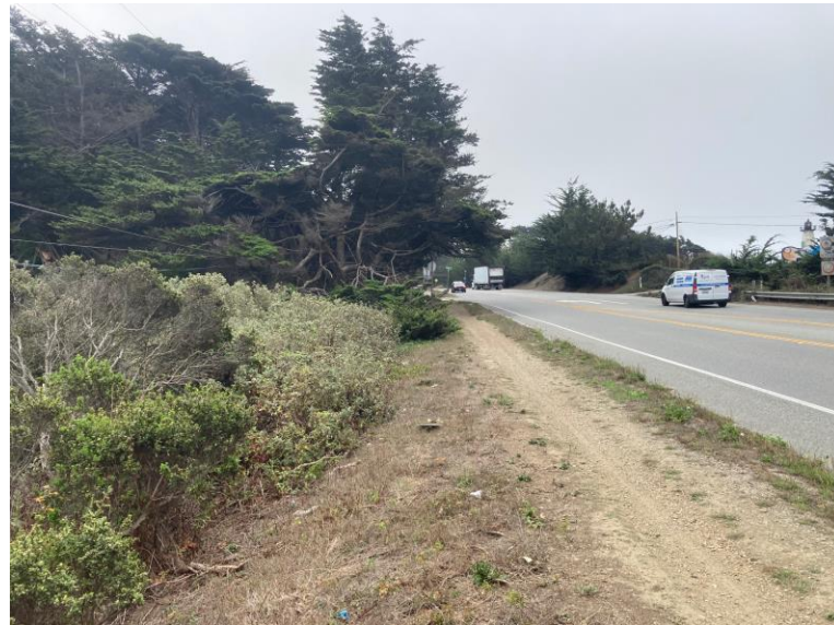
Northbound shoulder SR 1 near 16th St looking south
