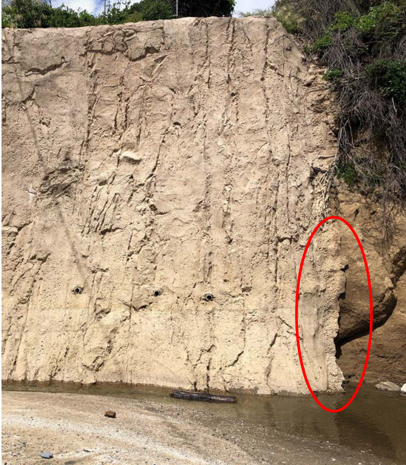
South end of North Wall
