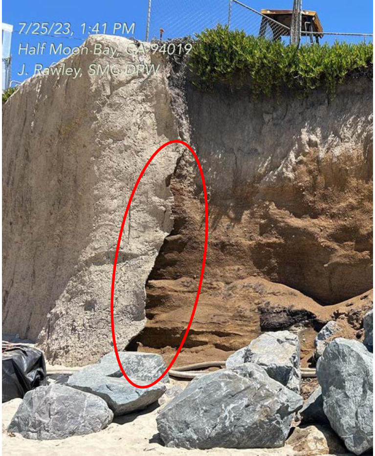
West end of South Wall
