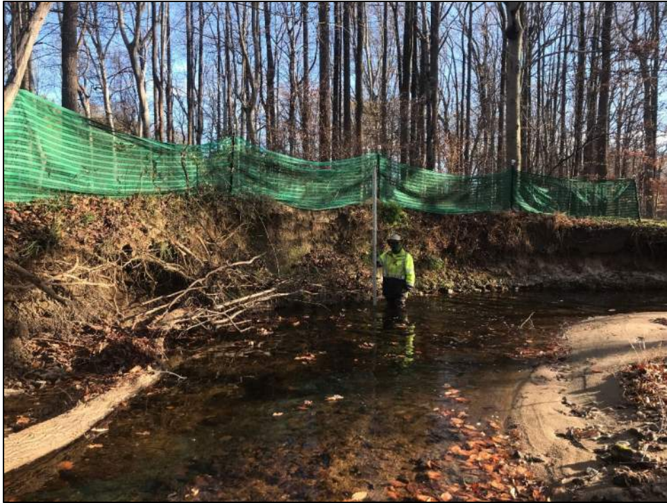
Photo 11: Reach 8A, looking downstream near Majors Ln, 8' actively eroding bank impacting nearby pedestrian path.
