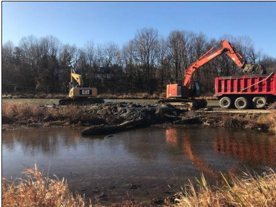
Photo 24: Reach 15C, looking downstream pond that ties into Lake Elkhorn, the pond is routinely dredged due to the high sediment load.
