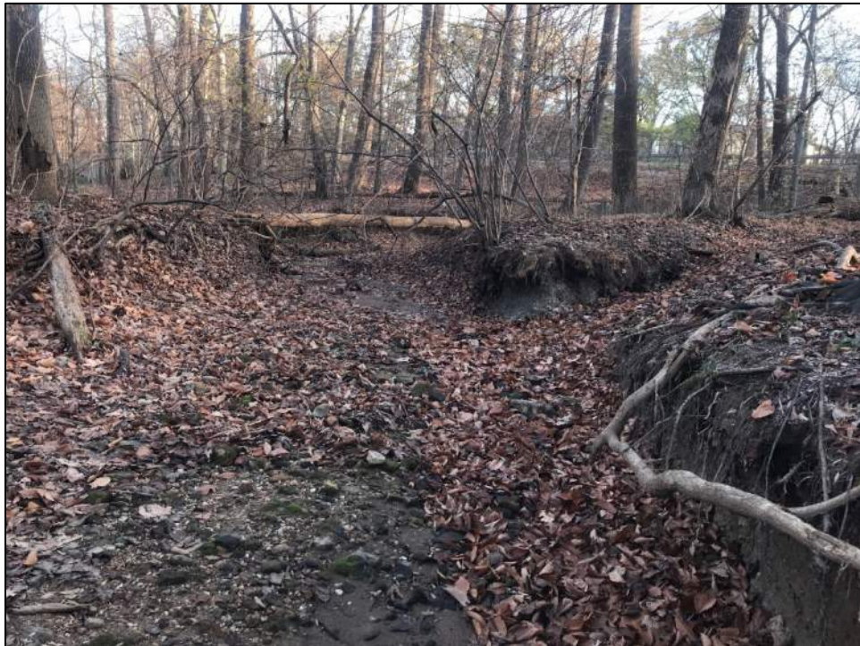
Photo 16: Reach 11, looking downstream near confluence with Reach 8A, 3' actively eroding bank with over widened channel.
