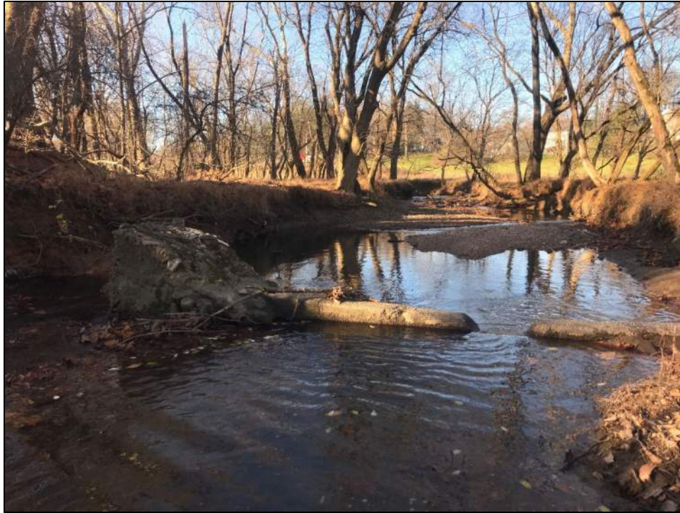
Photo 23: Reach 15C, looking downstream near Drowsy Day Drive, 4' actively eroding bank with exposed sewer line and over-widened channel.
