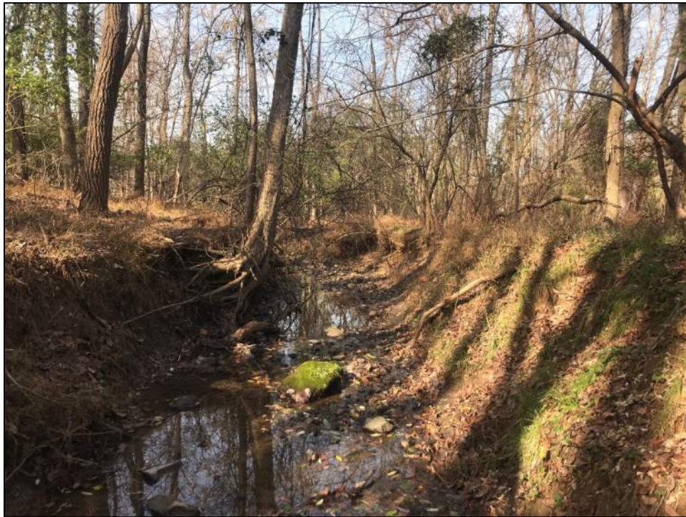
Photo 18: Reach 13, looking downstream near utility easement, 4' actively eroding banks. The riparian area contains a high concentration of invasive species.
