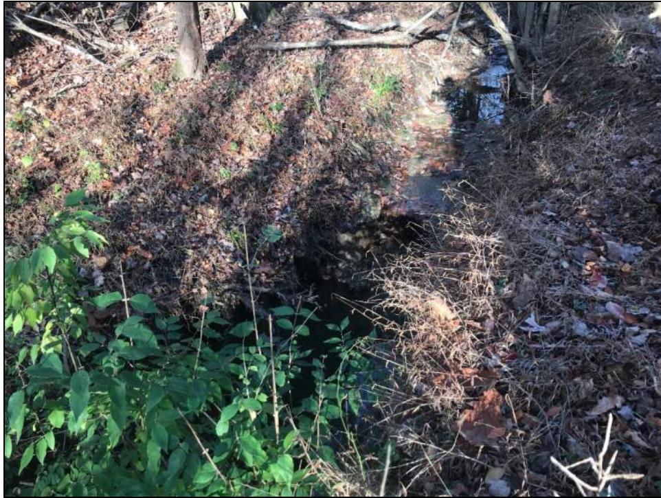
Photo 17: Reach 12, looking upstream near Stone Cloud Rd, 3' head cut.
