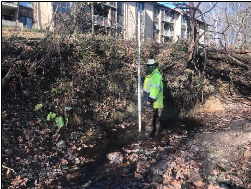
Photo 14: Reach 9A, looking downstream near Majors Ln, 7' actively eroding bank with minimal riparian vegetation.
