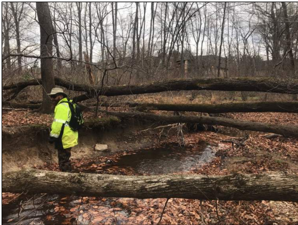
Photo 8: Reach 5, looking downstream towards Reach 3B, 3' actively eroding bank.
