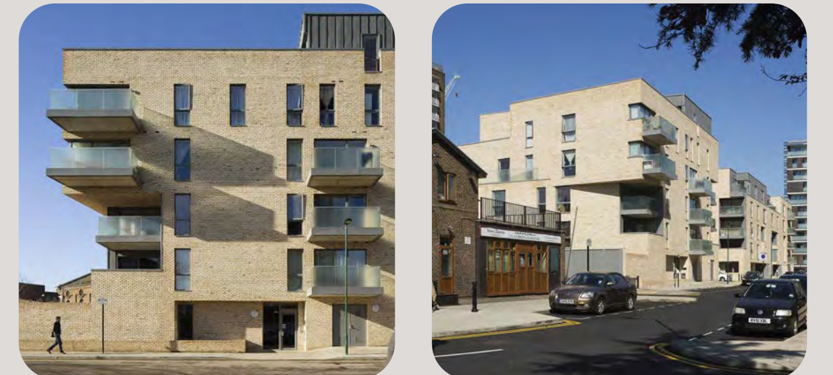
Hicks Bolton House MICA Single storey flats and double storey duplexes providing a distinctive view from Carlton Vale. Phase 1B
