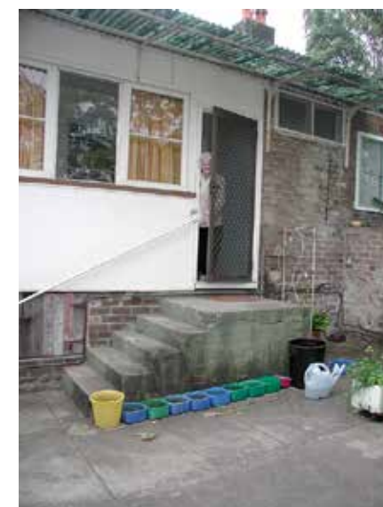
Peggy's rainwater-collection system, 2009
