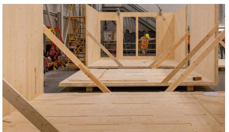
Our Mass Timber Model Home uses **mass timber pedestals** instead of truss or joist systems for subfloor support.
