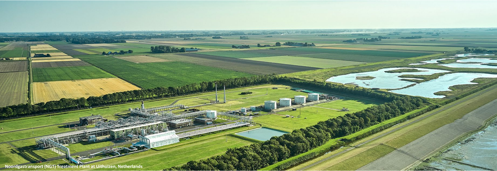
Noordgastransport (NGT) Treatment Plant at Uithuizen, Netherlands
