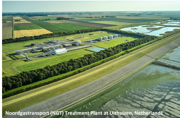
Noordgastransport (NGT) Treatment Plant at Uithuizen, Netherlands
