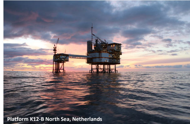
Platform K12-B North Sea, Netherlands
