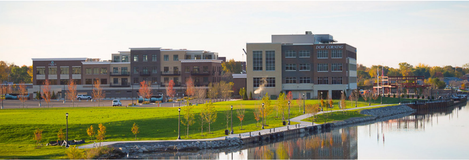
The Uptown Bay City development provides a glimpse into possibilities for mixed-use development on Consumers Energy’s Saginaw River frontage. Setting mixed-used structures back from the river’s edge with a buffer of landscaping and paved pedestrian pathways provides a model for multiple site uses and user groups to co-exist.
