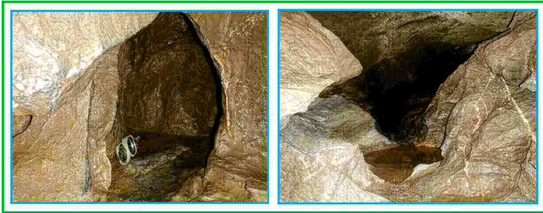
Figure 6. Solution conduits in the Onondaga limestone can rapidly transmit contaminants with little or no dilution and cleansing, including through finger-sized conduits. This is analogous to open pipe flow, resulting in the most vulnerable of hydrogeologic settings.
