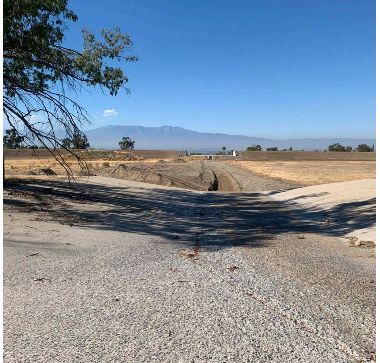
Oak Street Basin at Chase Drive
