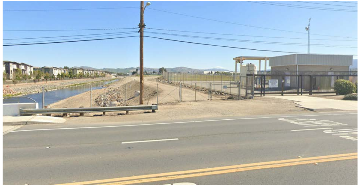
The top ranked Public Safety Way trail connects Lincoln Avenue to North Cota Street via a flood control channel
