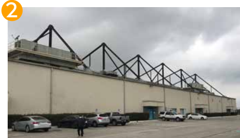
Aircraft Maintenance Hangar (1972-1979)
