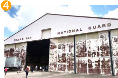
Texas Air National Guard Hangar (1961)
