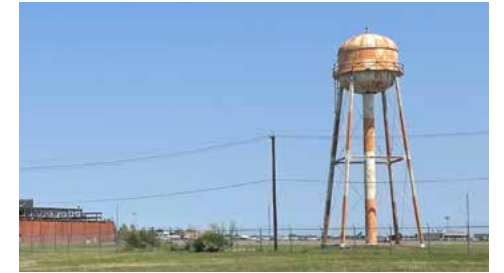
DNAS Water Tower (1941)
