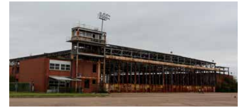
Dallas NAS Maintenance Hangar (1941)
