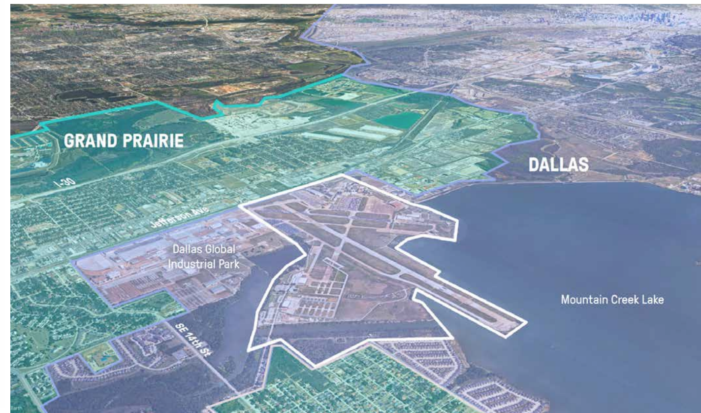
The Hensley Field site (white border) with Downtown Dallas in the distance.
