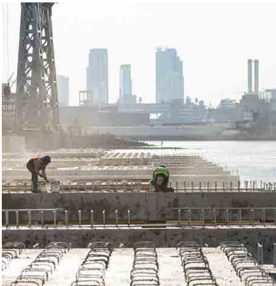
Constructing Domino Park, Brooklyn
