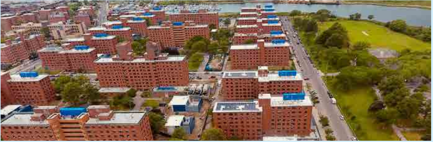
Generators and solar panels installed on the roof of each building of Ocean Bay Bayside Apartments in Arverne, Queens (Credit: NYCHA)
