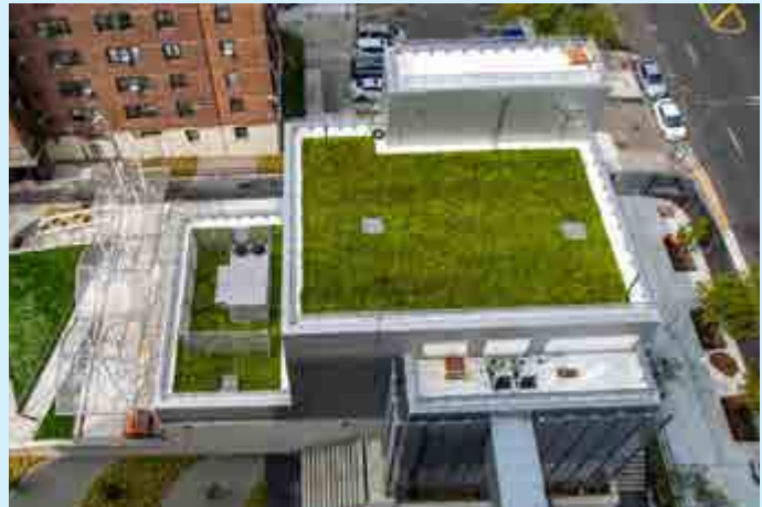
Elevated boiler building, with shade structures, community space, green roofs, and site improvements serving multiple buildings at Coney Island Houses in Brooklyn (Credit: NYCHA)
