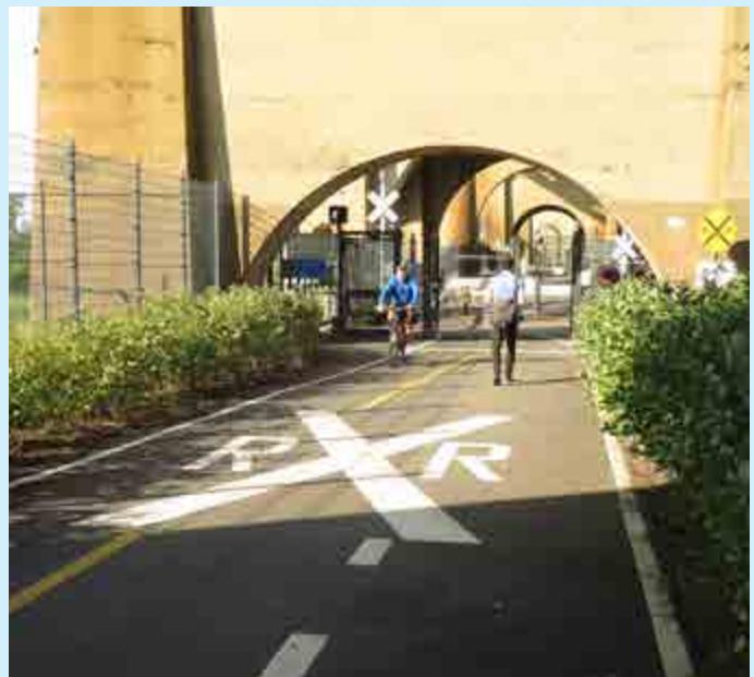
Randalls Island Connector Credit: NYCDOT
