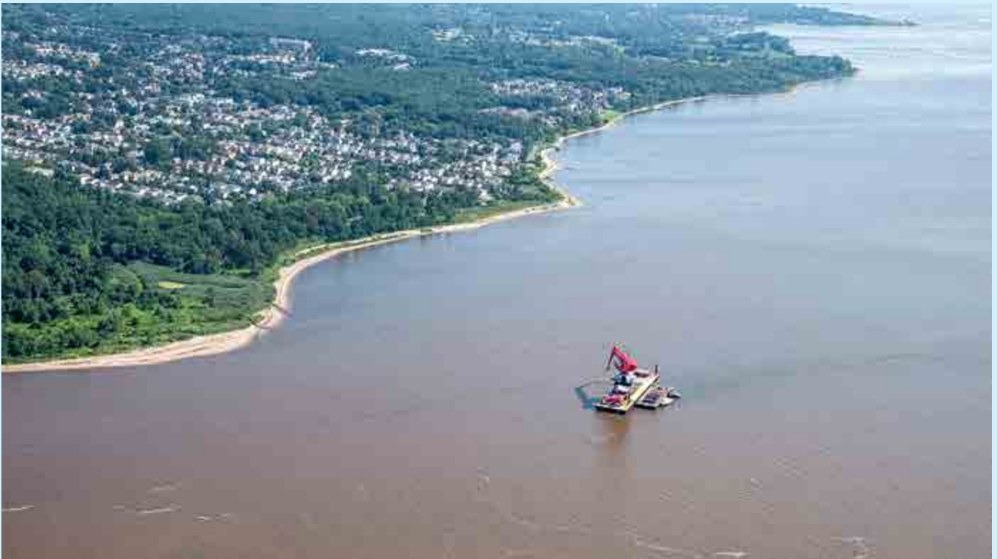
Above: Living Breakwaters Construction, Staten Island
