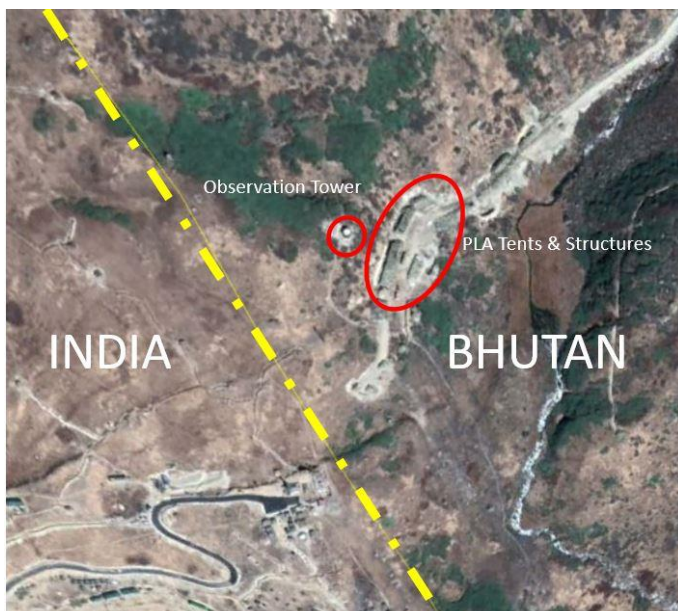
Figure 14. Corresponds to site A in Figure 7. Concrete structures and tents are clearly visible on the Chinese side.
