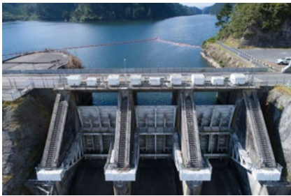
Matakina Dam, Bay of Plenty
