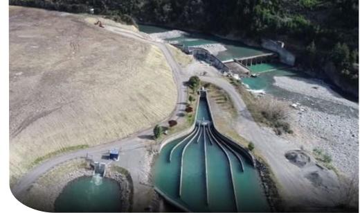
New Branch infiltration gallery with discharge into the Argyle Canal
