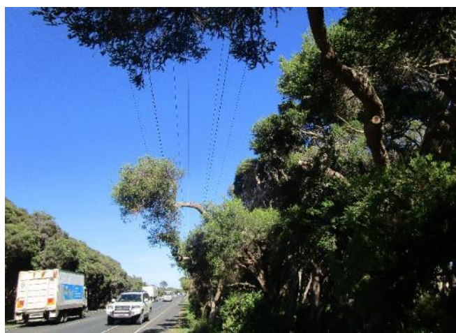
Power line pruning impacts
