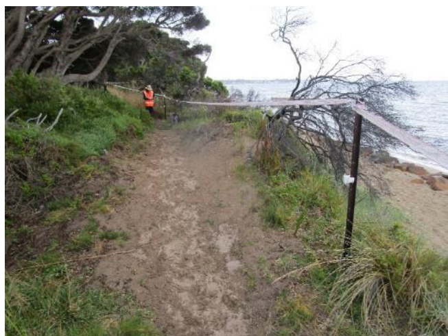
Temporary fencing been installed to try and manage foreshore erosion due to walking track and vegetation impacts
