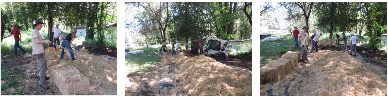
Fig. 9. Final treatment of remaining untreated contaminated soil
