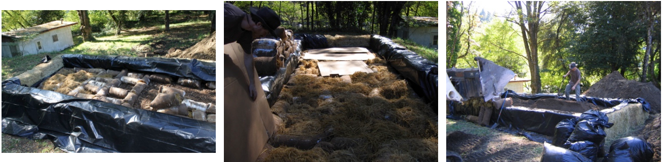
Fig. 4. Inoculated burlap sacks being laid out and layered with contaminated soil
