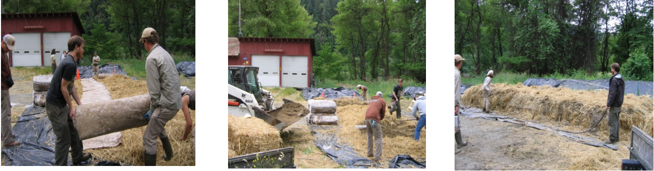
Fig. 6. Layering straw, inoculated burlap, and contaminated soil into piles
