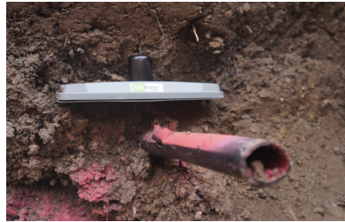
InfraMarker underground tag placed over water pipe near a catch basin
