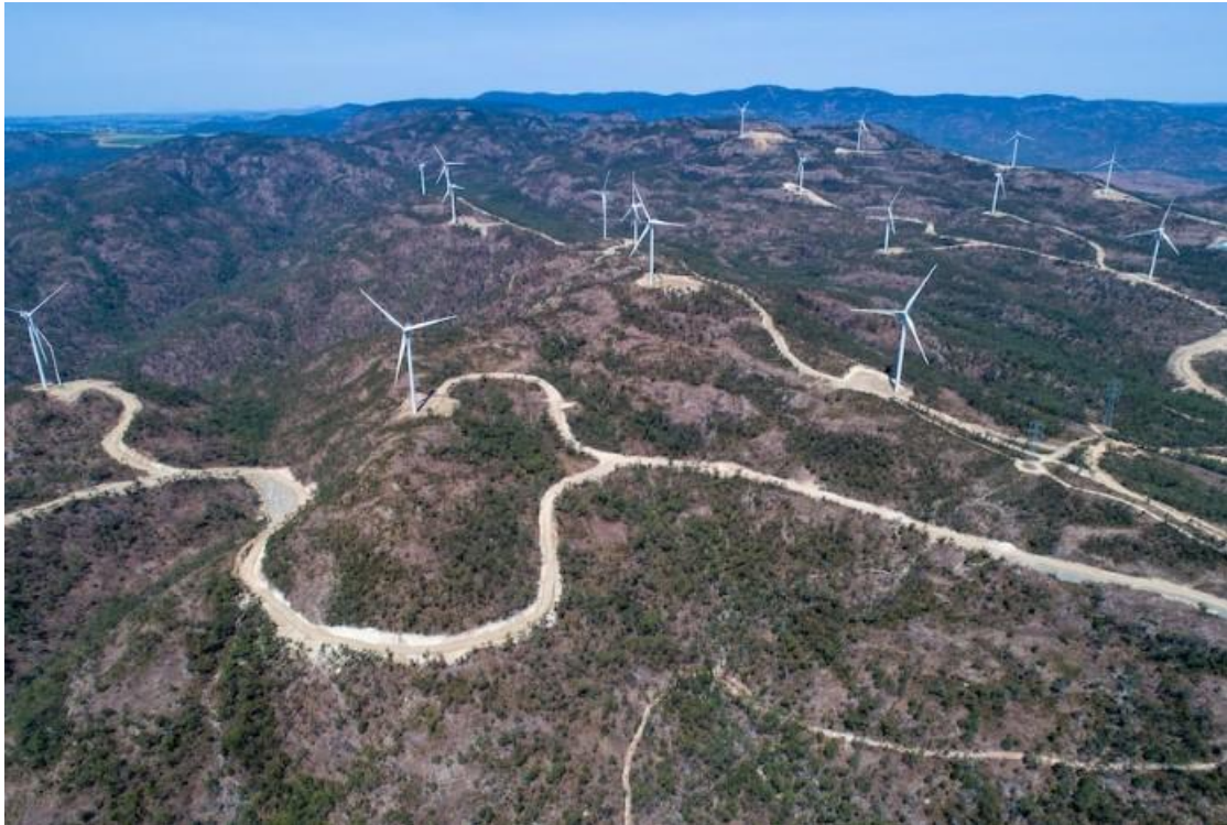
Figure 3. Fragmentation at the Mount Emerald Windfarm. Note that the proposed Chalumbin, Upper Burdekin and Mount Fox windfarms will have much taller turbines and therefore much larger pads and considerably wider roads. Photo Steven Nowakowski.
