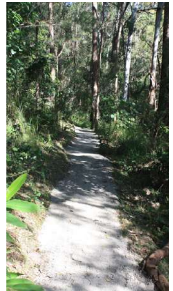
The top sixty metre section completed with compacted road base surface and cross fall drainage
