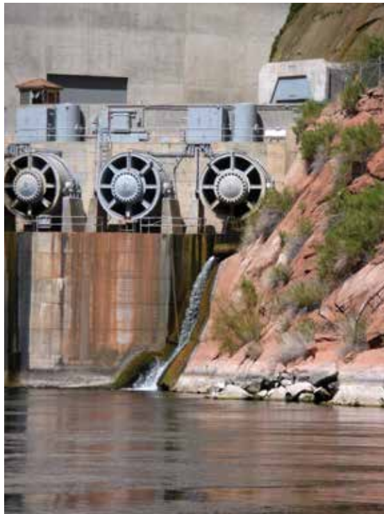
Glen Canyon Dam Jet Tubes photo by Lynn Hamilton
