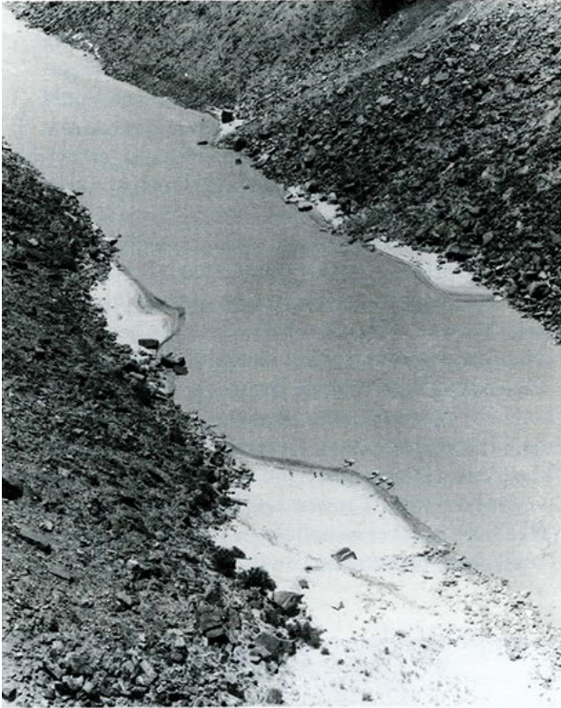
A. (July 1956). A Mexican Hat Expeditions is stopped for lunch at the large separation bar downstream from Jackass Canyon. Driftwood lines the beach, separating the "Pyramid Rock" (above) from the "Turret Rock" (barely showing below). (Tad Nichols, courtesy of the photographer).
