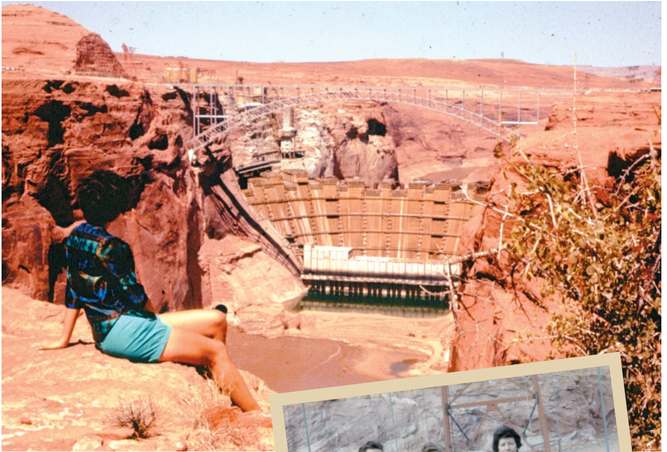
Pat Diamond, watching the dam go up.
