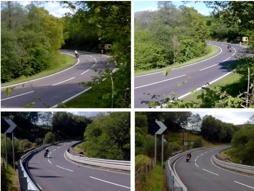
Figure 7: Changes in road position (left-hand images = without PRIMEs installed, right-hand images = with PRIMEs installed)
