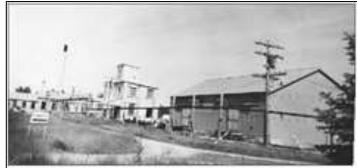
By 1934, seventeen buildings had been constructed and the plant employed 30 people with a monthly payroll of about \$2,000. Many safety features were incorporated such as the 80-ton sand-filled barricades erected around the buildings to direct any explosion straight up rather than side-ways. Employees caught ignoring safety rules were fired on the spot.
