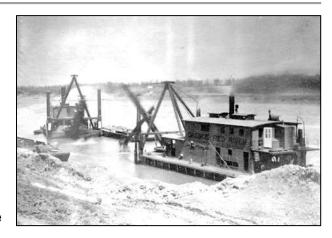
In more recent years, dredges involved a more modern suction system where a snorkel like tube with cutting bits on the end would dig into the river bottom and then with water, pump the sediment through a long pipe to the edge of the river bank.
