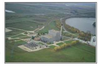
2002 the plant underwent a \$30 million conversion from coal to natural gas reducing emissions by 46%. The 2 gas turbines have a capacity of 12,500 kw per unit.
