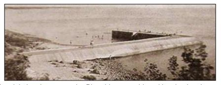
deflect the ice and strong wave action to help minimize damage to the Pier; this was achieved by slanting the siding of the Pier.
