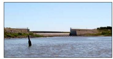
Over time portions of the floodway were compromised so in 2014, a \$627 million floodway expansion program was completed which involved rebuilding the outlet at Lockport; improvements to the Inlet Control structure, raising train and highway crossings and increasing the floodway capacity to allow a flow rate of 4,000 cubic metres (140,000 cubic feet) per second, the estimated level of <u>a one-in-700 year flood event.</u>
