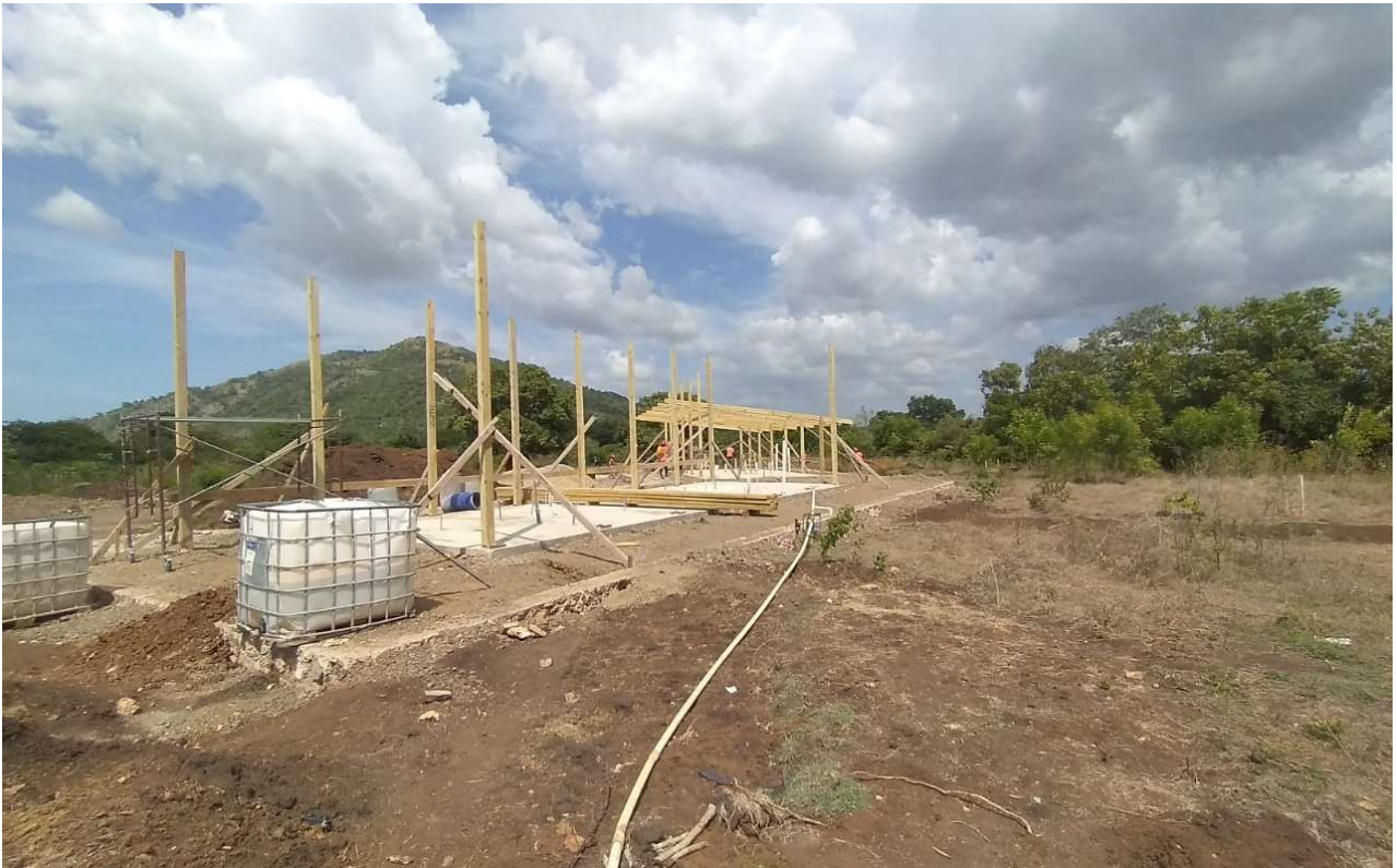
Photo 6: Timber assembly underway.
