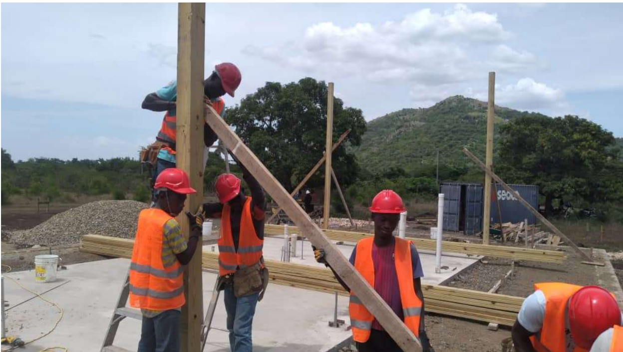
Photo 2: Assembly started with positioning corner columns.
