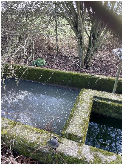
Figure 2-3 - Oil interceptor located close to the southwest boundary (Sculpins Lane).
