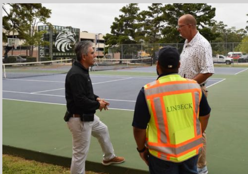
Mr. Enrique Ambrosio, assistant facilities director, and Mr. Carter Metclaf, project coordinator, discuss the demolition of the tennis courts adjacent to parking lot outside the high school. The parking garage will be instrumental as more construction gets underway on campus.
