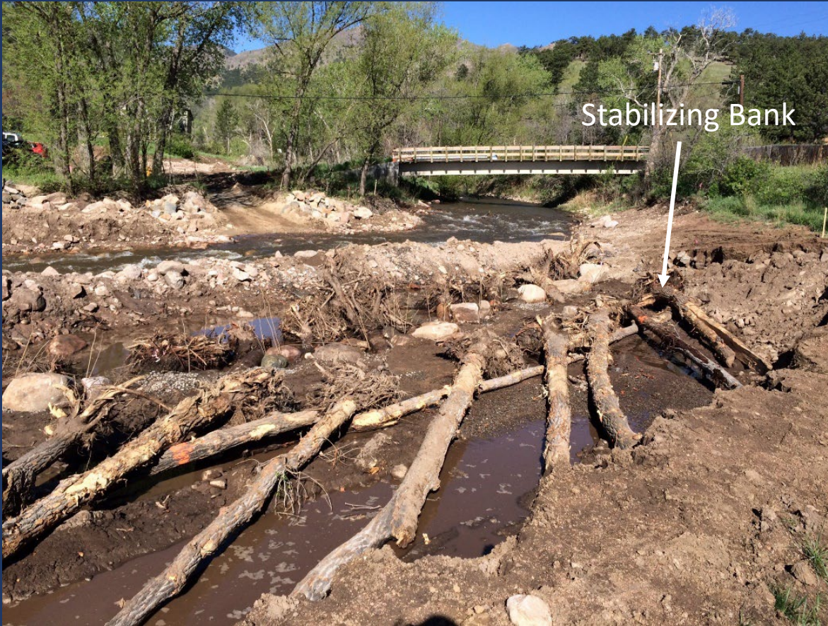
Wood Revetment During Construction, Fall 2016
