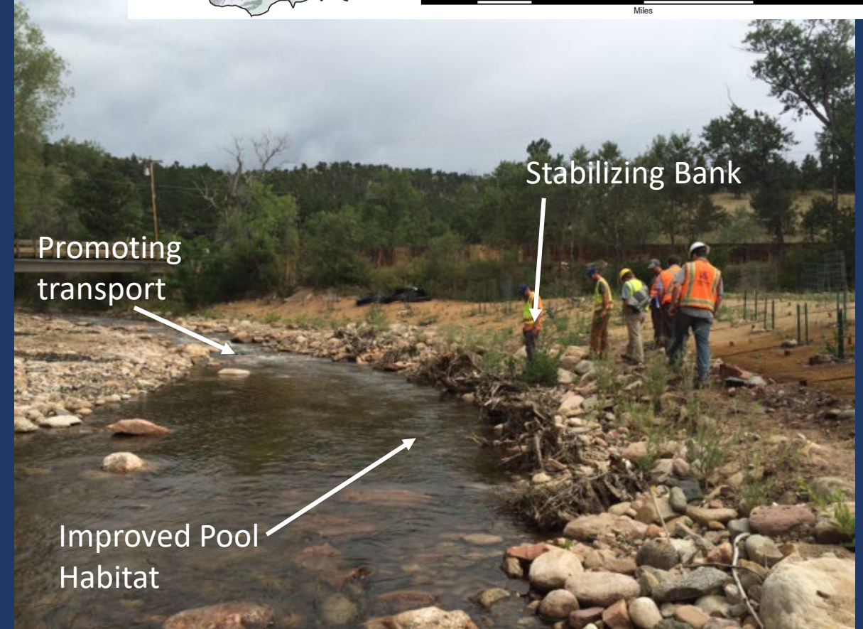
Post-Restoration Wood Revetment, Summer 2017
